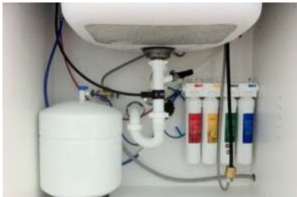
Typical Under Sink Installation
