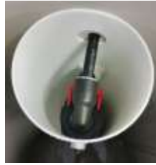
Brine Well with safety float and air
