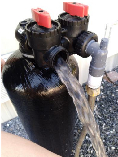
Flushing the carbon with garden hose attachment. (Part number: F-FLUSH.)
