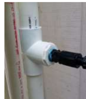
Chemical injection fitting. Install directly before the contact tank.
