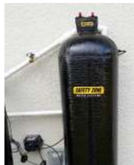
Contact tank for Hydrogen Peroxide. (No bottom drain)
