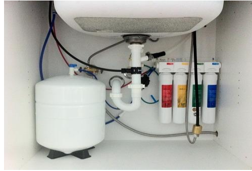
RO-4 system with quick change cartridges. (Storage tank included.)
