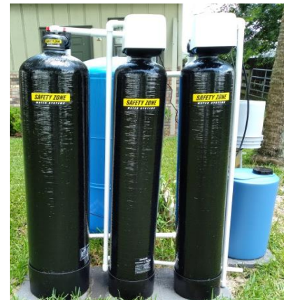
System with 13x54 contact tank. (Be sure to use weather covers outdoors.)
