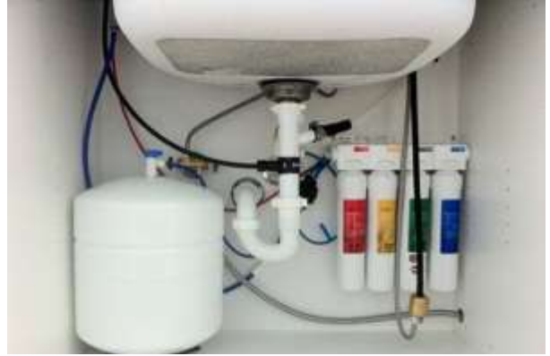
Typical Under Sink Installation
