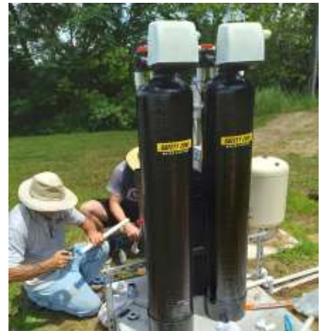
Weather covers are required in outdoor installations. (See above.) Part Number: WC-SS-W
