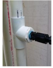
Chemical injection point before the contact tank.
