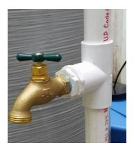
Install a hose bib after contact tank for chemical testing.
