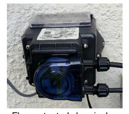
Flow actuated chemical pump. No flow switch needed. Connects to relay in softener valve.
