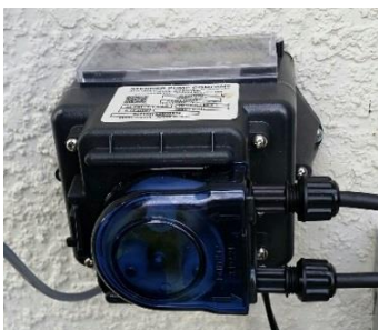
CFP-ROLLER Flow actuated chemical feed pump.
